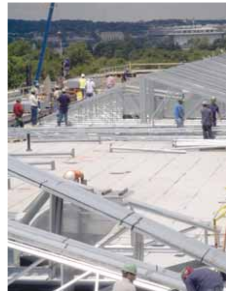
Rebuilding the Pentagon
