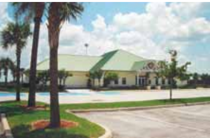
PGA Headquarters, FL
